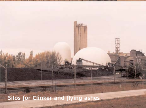
Silo for Clinker Capacity 40.000 Tn.
